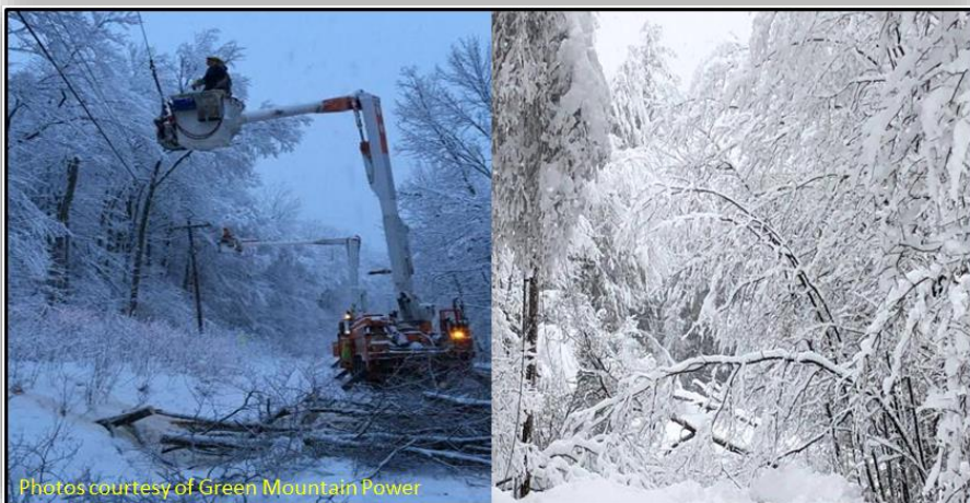
Figure 4. Pictures showing the damage from the heavy wet snowfall. Photos courtesy of Green Mountain Power.
